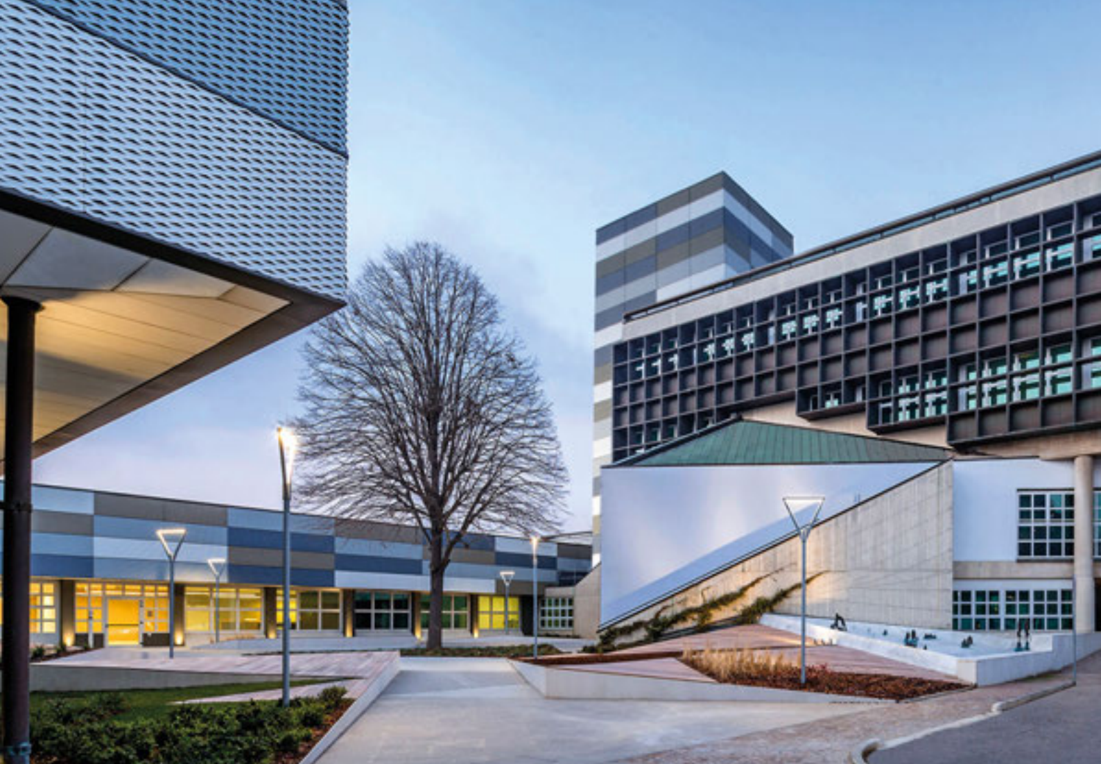
Worklife Innovation Hub, Casalecchio di Reno, Bologna, Italy - Open Project © Ph. Diego De Pol
